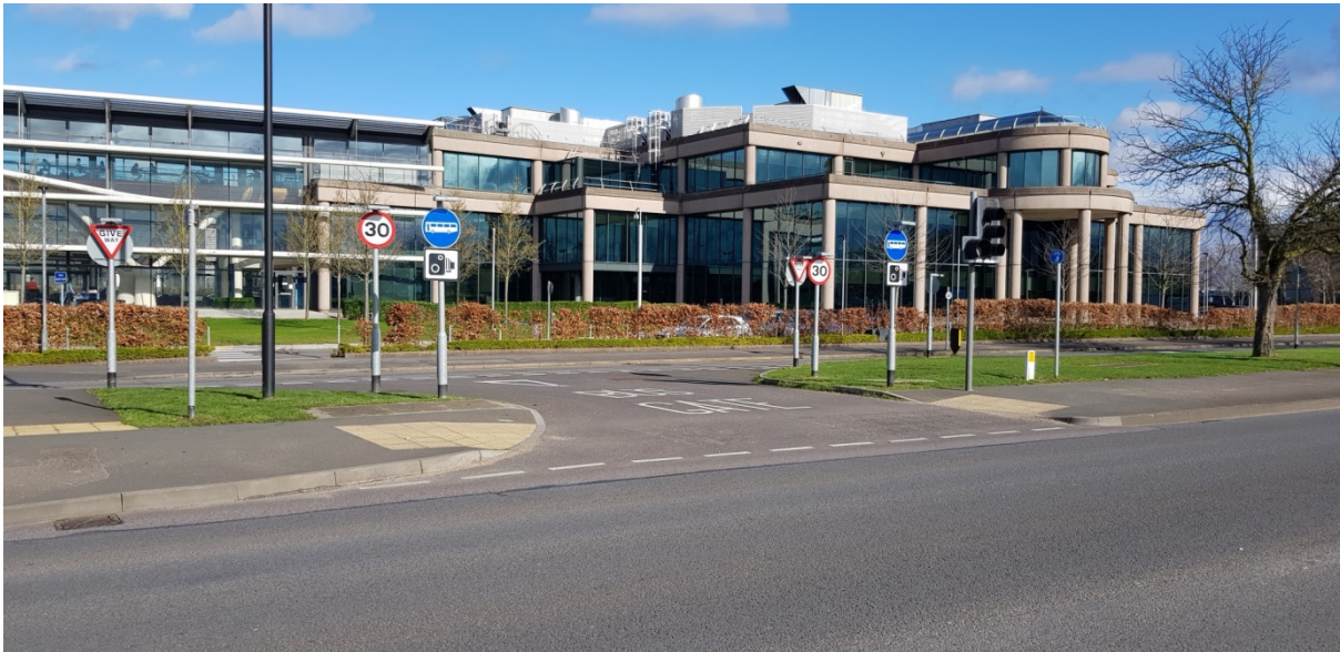
Image 1: Telefonica/O2 – accessed via the SMaRT bus gate leading onto Bath Road Service Road North
