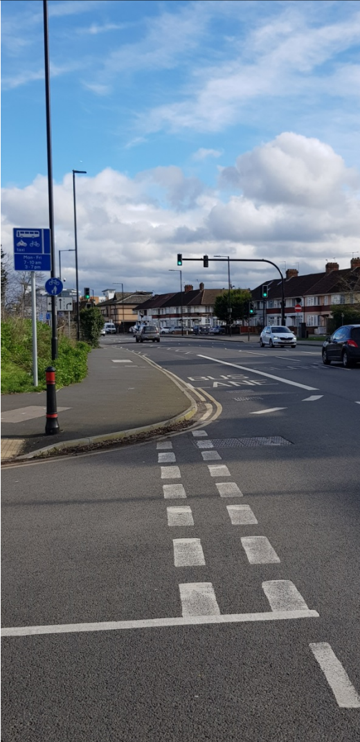
Image 3: Junction of Bath Road Service Road North and the A4/Bath Road
